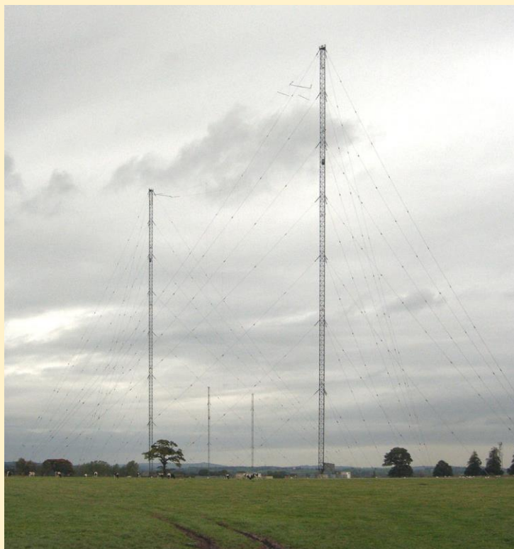
Picture: Droitwich 198kHz t-antenna, between the 213m tall masts.
